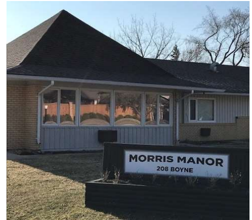
(12) The Morris Manor Limited - Upgrades & Improvements to the look and function of the Morris Manor.
